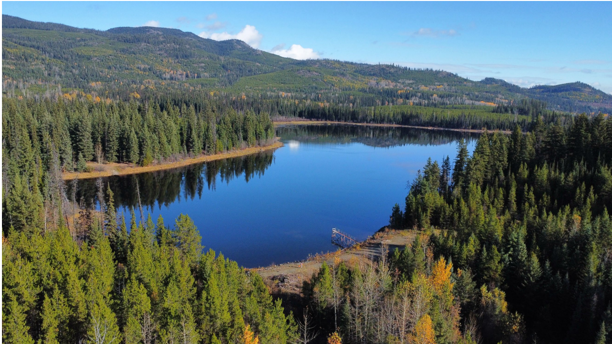
FIGURE 2-1. LEONIE DAM DRONE PHOTO (INTERIOR DAMS, 2024)
