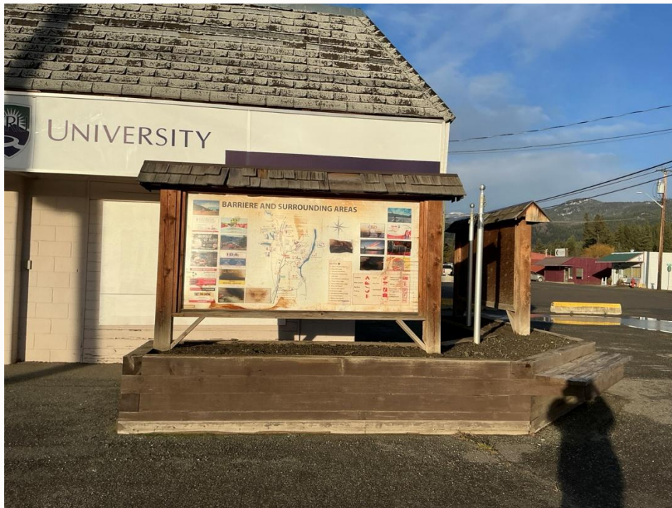
Existing information kiosk with worn and aging signage
