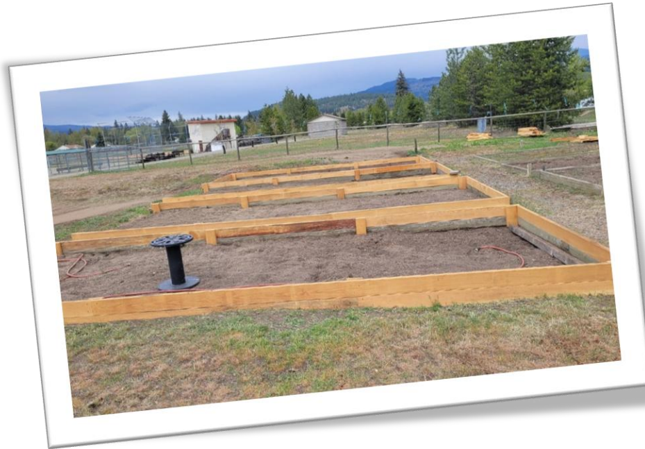
Newly replaced garden plot frames
